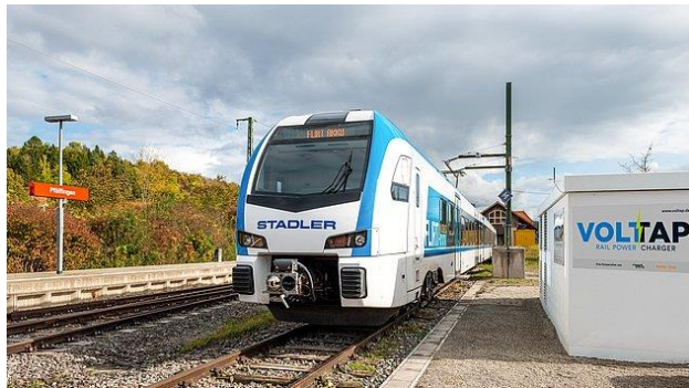
October 2021 Tübingen VOLTAP – Furrer+Frey 15/25 kV 50 Hz – 2 x 1,2 MVA © Stadtwerke Tübingen
